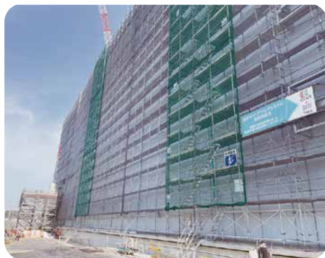
(仮称)NRT10新築工事
